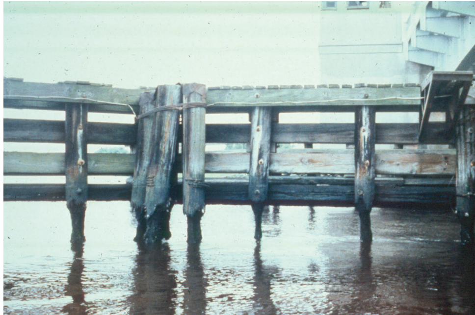
Figure 10.2.55 Timber Fender System
