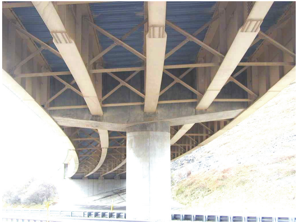
Figure 10.2.12 Integral Pier and Pier Cap
