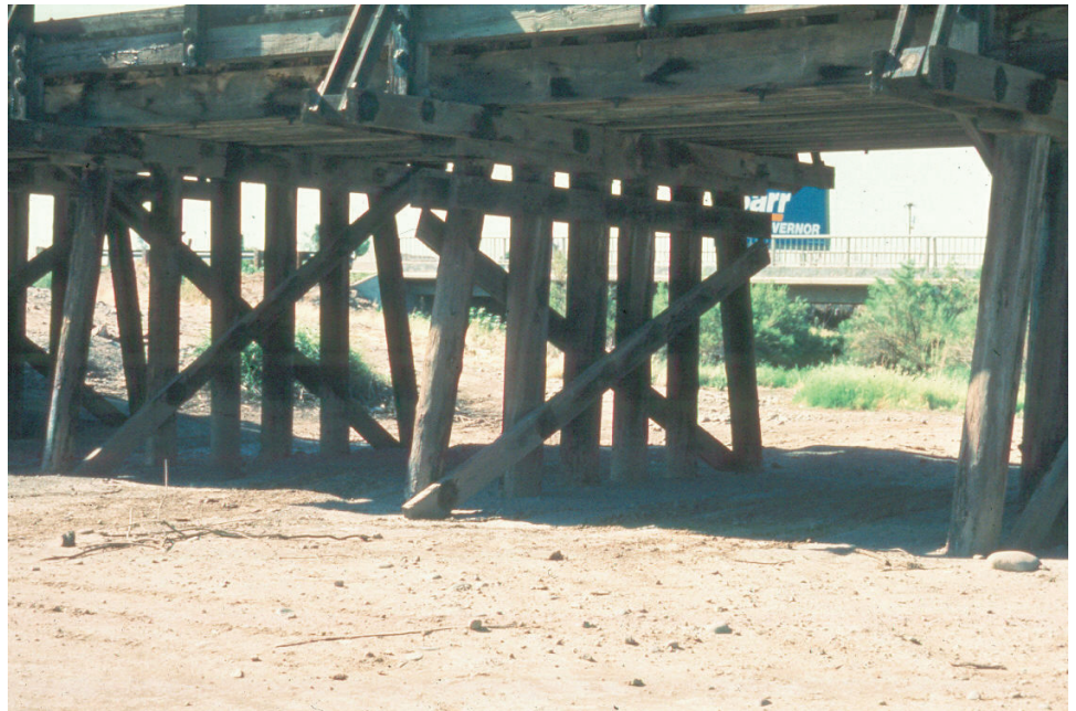
Figure 10.2.16 Timber Pile Bent
