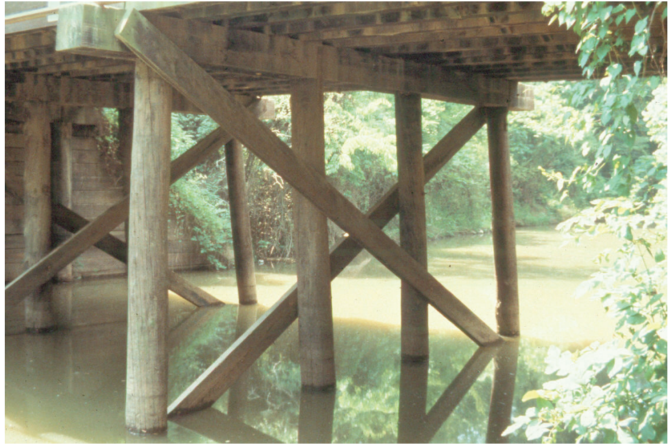
Figure 10.2.46 Timber Bent Columns in Water
