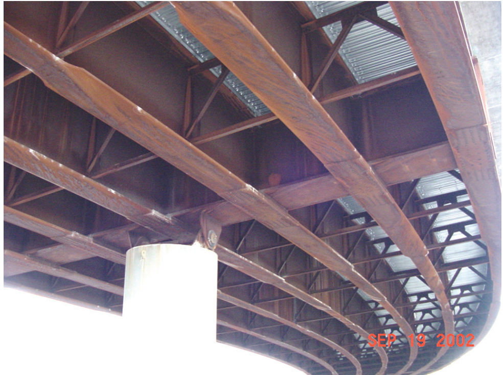
Figure 10.2.10 Integral Pier Cap
