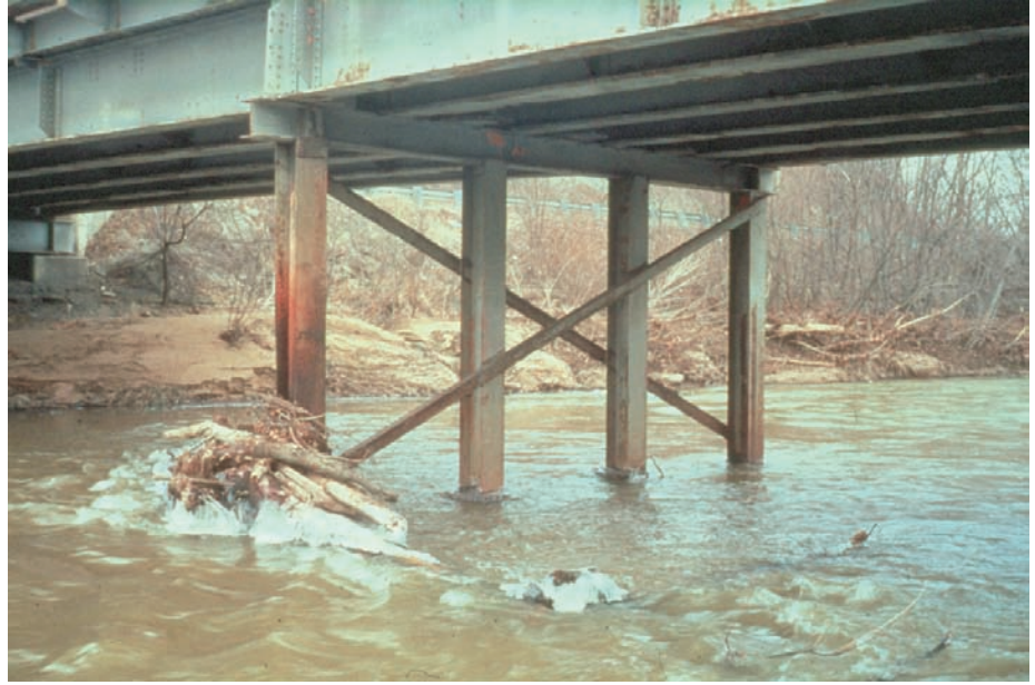
Figure 10.2.41 Corrosion and Debris at Steel Pile Bent
