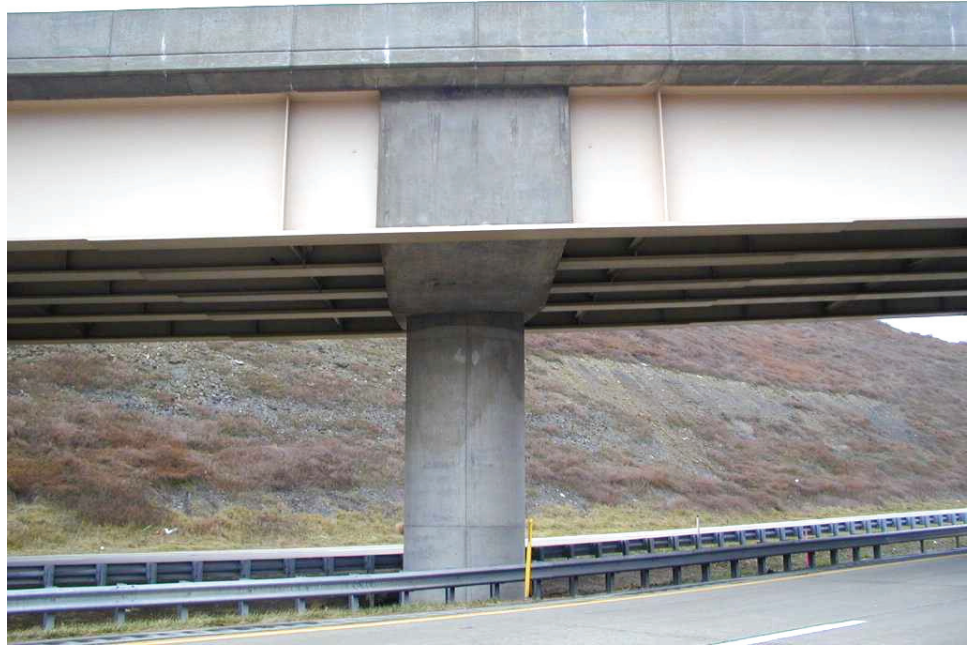
Figure 10.2.11 Integral Pier and Pier Cap
