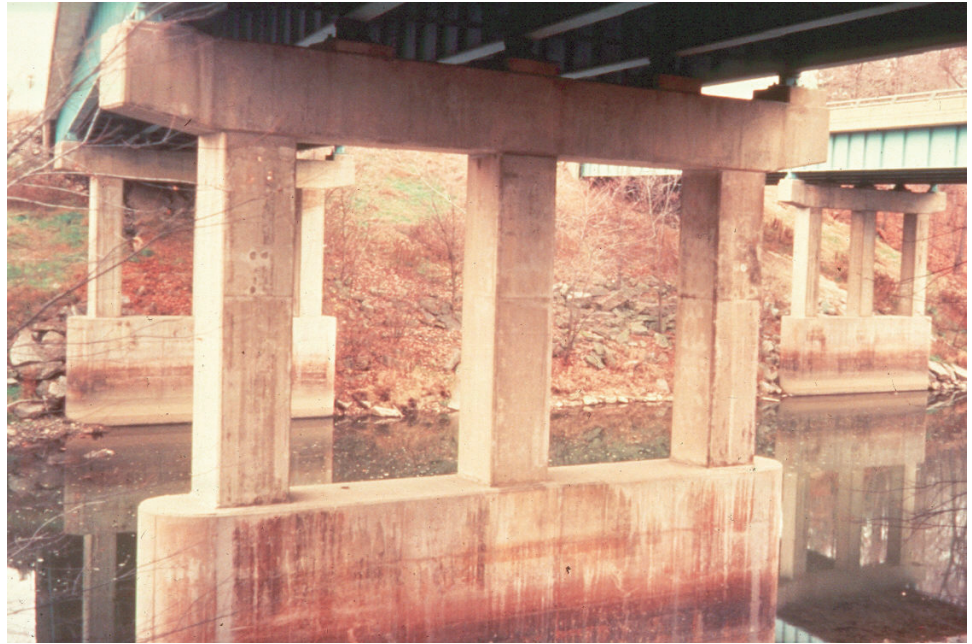
Figure 10.2.25 Collision Wall
