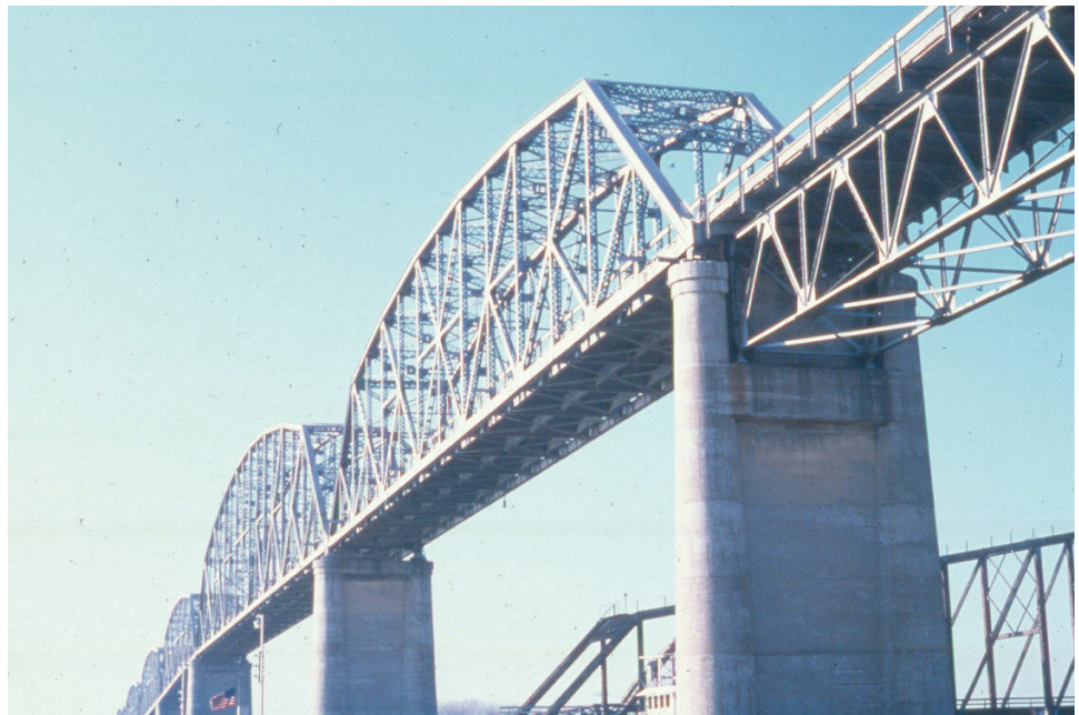
Figure 10.2.5 Column Pier with Web Wall
