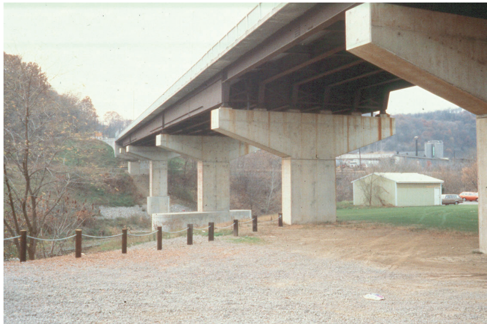
Figure 10.2.7 Cantilever Pier
