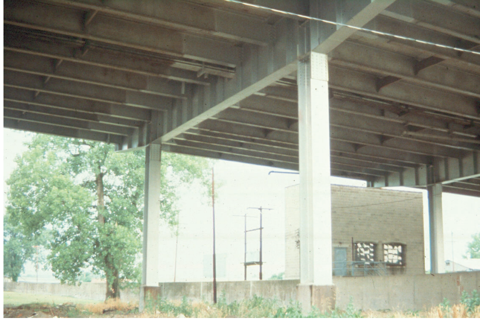
Figure 10.2.43 Steel Column Bent with Cantilever
